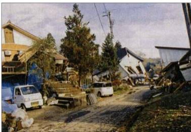
After the earthquake
