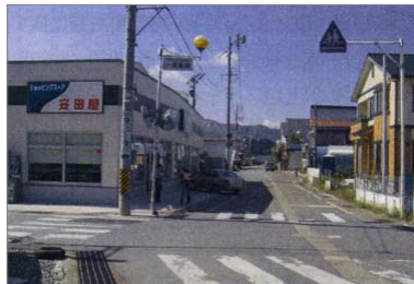
At the end of the restoration process
