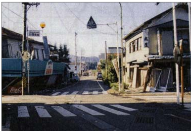
After the earthquake
