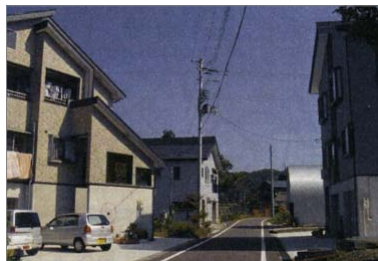
At the end of the restoration process
